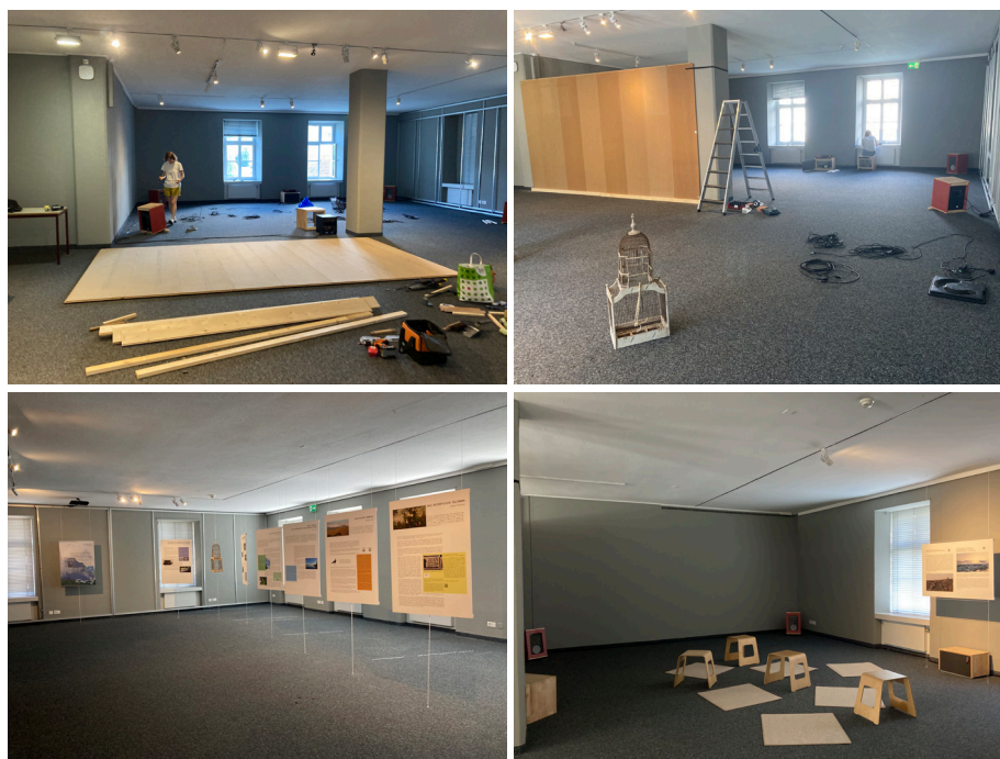
Fig. 4–7: Dividing the exhibition room with a temporary wall and mounting the audio installations and posters, Photographs by Helena Simonett, September 2022.
