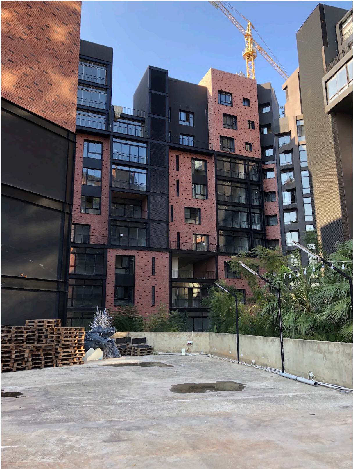
Figure 5 : UPARK 128g; external view from Station Beirut's rooftop. Image courtesy of the author, Photographed by the author.
